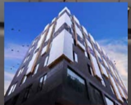
A commercial complex
